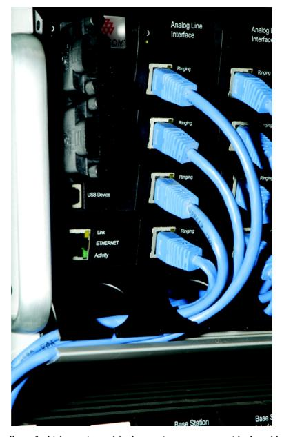
Figure 1-13 Harnessing cables to the side and out.
